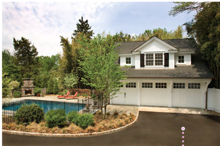
A three-car detached garage was redesigned and rebuilt to include an exercise room and bathroom for the nearby pool (photo by Tom Grimes).
